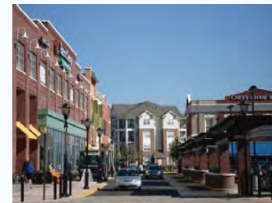
Successful plans define core and residential areas, and the transitions between them.
